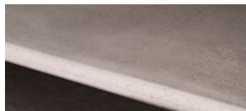
Reinforced concrete plate
